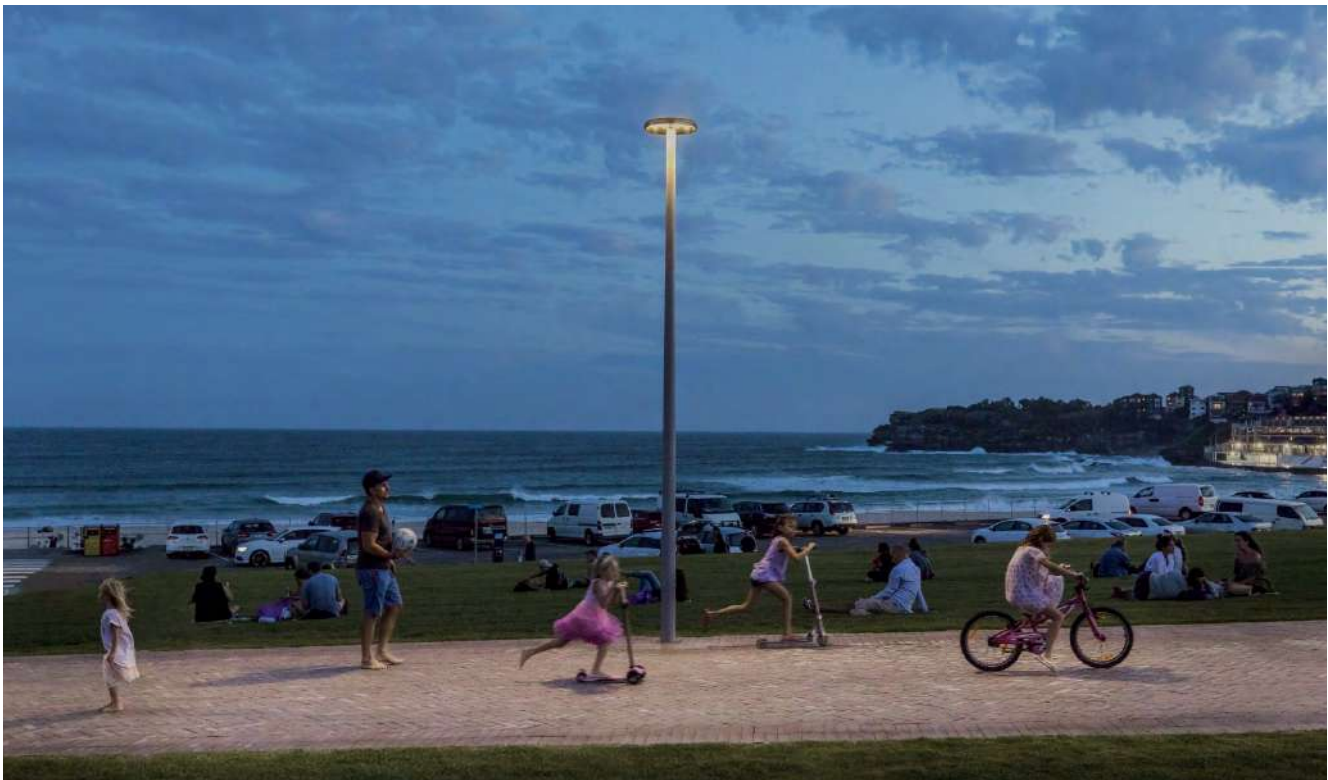
Shown in this example are RMT320 [S60] Two-sided Streetlighting distribution
