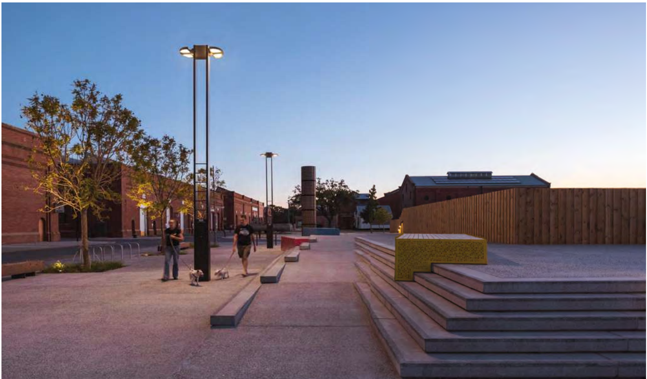
Shown in this example are RMC320 [S60] Streetlighting distribution
